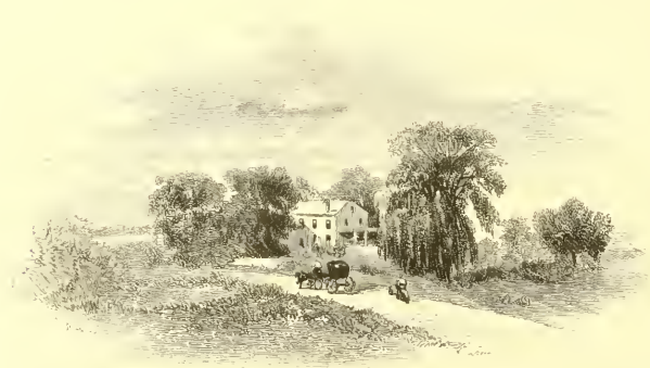
OLD HOUSE BY RESERVOIR.
